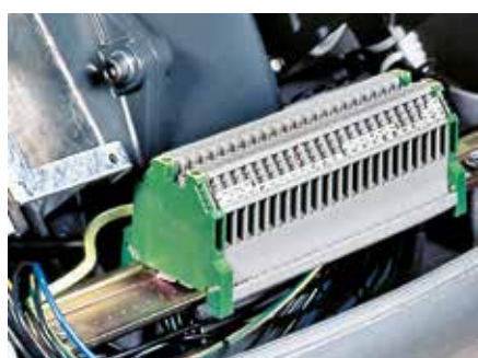
Example of the terminal board for electrical connections for the RS 70-100-130-190-250/M models.
