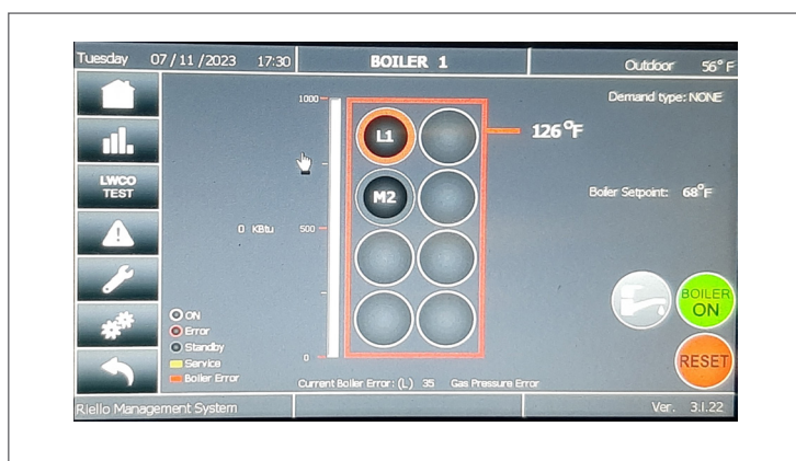
Fig. 44 Boiler Screen
