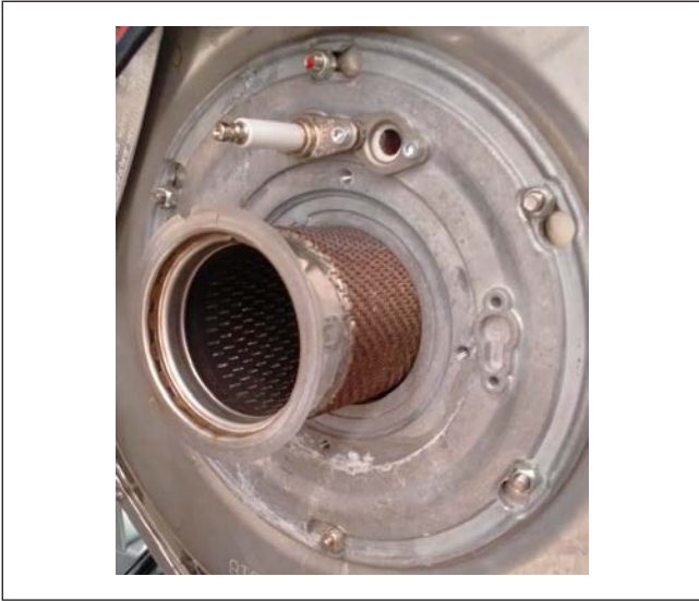
Fig. 7 Burner lead
